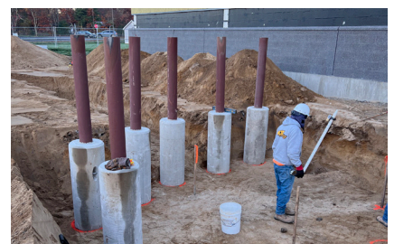
Above: Site bollards being installed at service areas.
