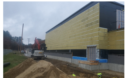
Above: Insulation installation at hardy panel back corner of gymnasium.
